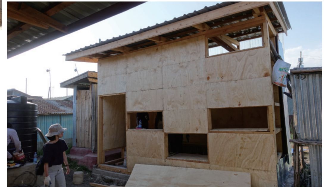
①② exterior wall installation ③④⑤ interior wall installation
